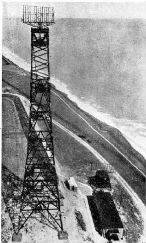
Rotating beam arrays used at CHL stations. The 185-ft. tower is used at sea level and the 20-ft. gantry shown on the right is for installation on cliffs.
